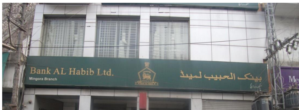
Figure 5.2 AL Habib Bank
